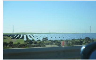
Vena Energy selects Doosan GridTech as EPC for 41MW Taillem Bend 2 BESS
